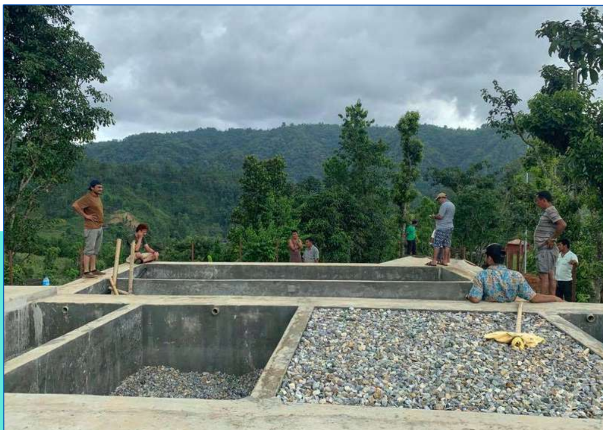
Construction of a Slow Sand Filter, Baglung
